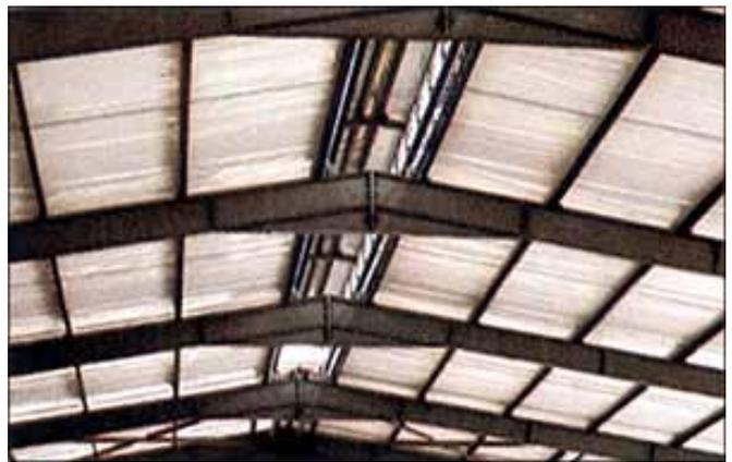
Thermal insulation and vapour barrier for roofing.
