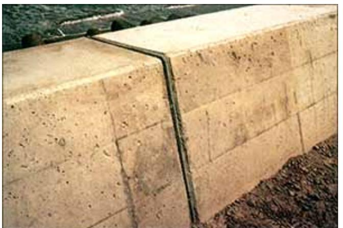
Joint filler for civil and building works, as the foam can accommodate expansion and contraction of the works. The foam does not absorb water during wet construction.
